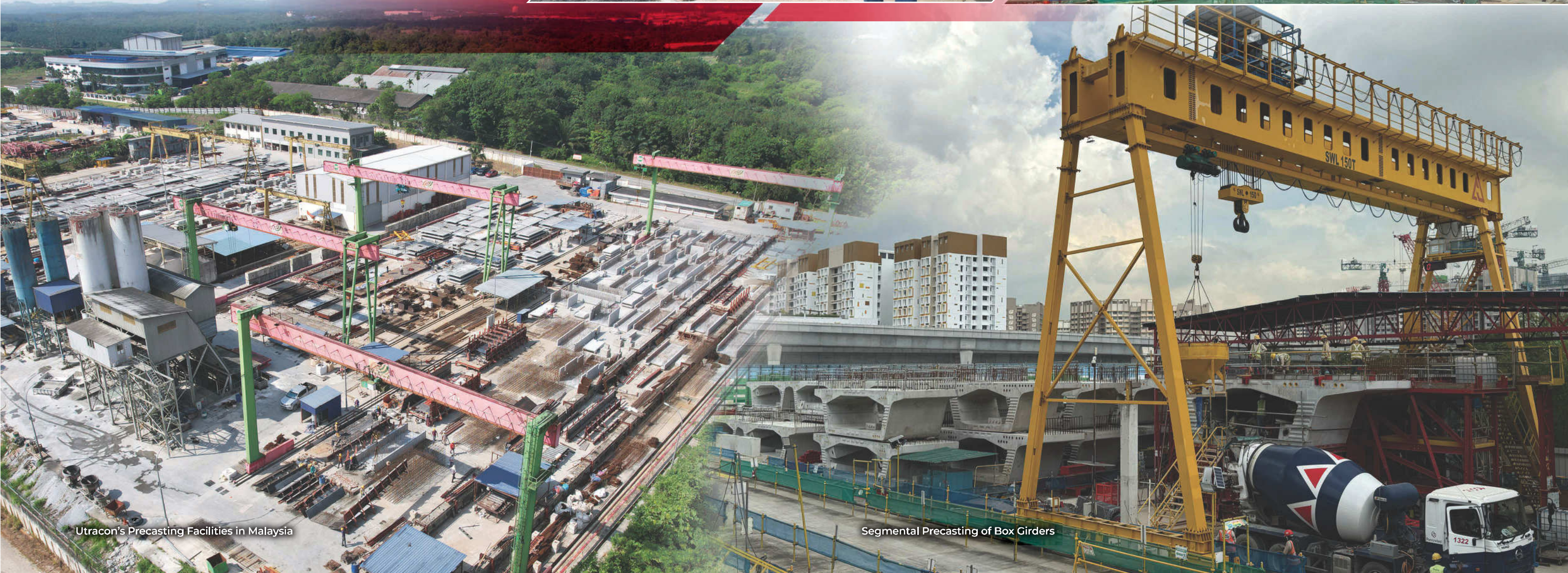
Segmental Precast Girders
