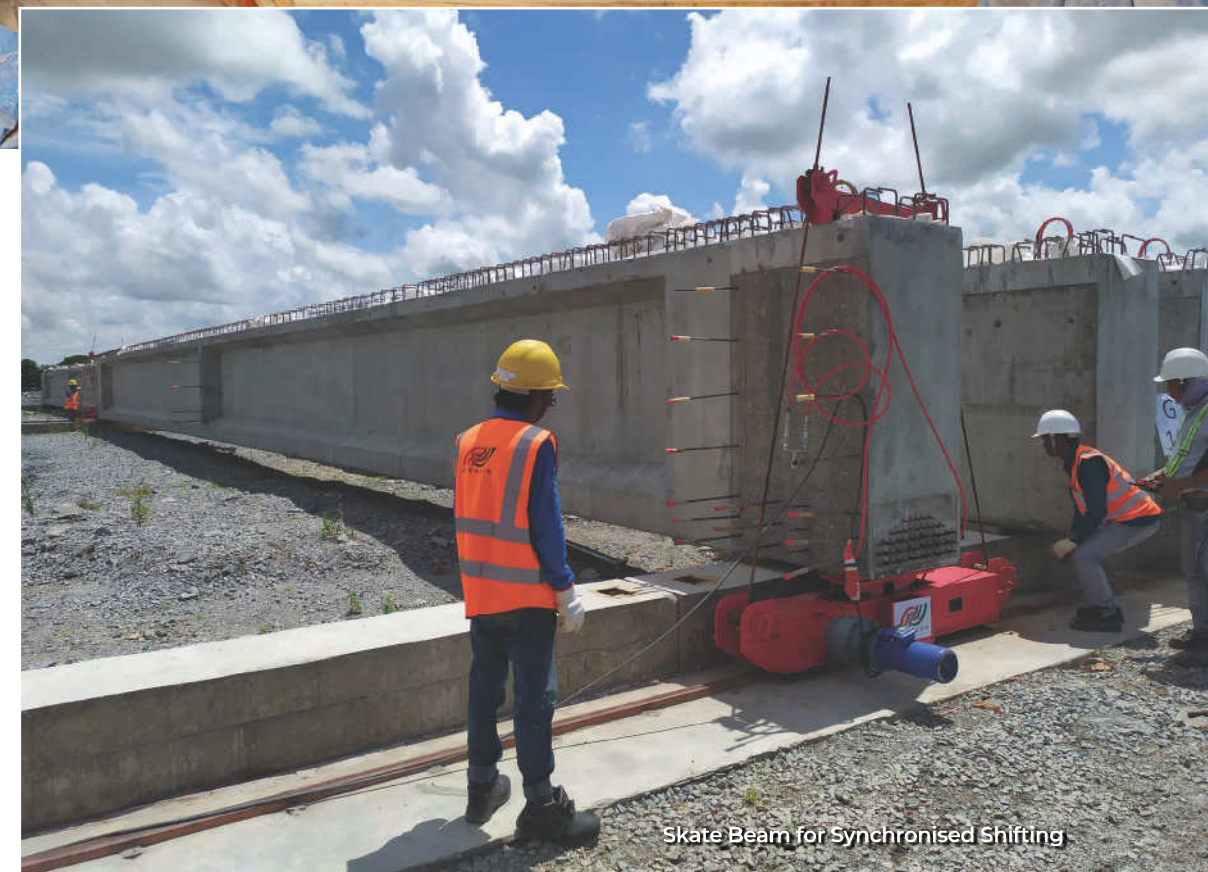
Computer-controlled Incremental Launching System
