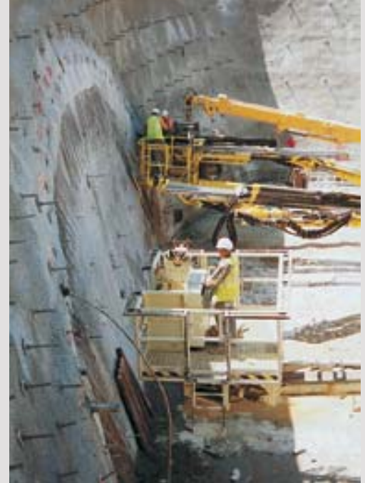
The drill platforms were fixed to telescopic arms on the upper levels
