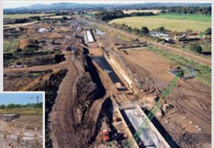
View of the 1.6 km long track section
