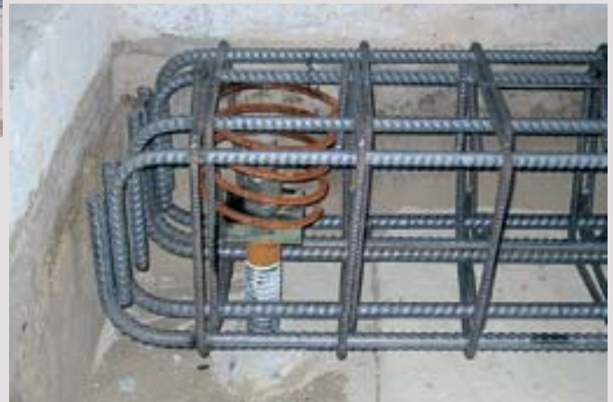
Detail view of GEWI® Pile head (compression)
