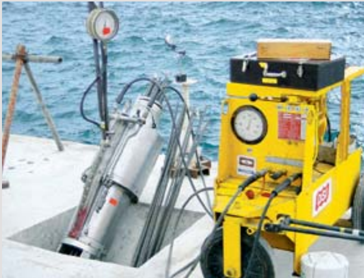
Tensioning of the DYWIDAG Multistrand Anchors
