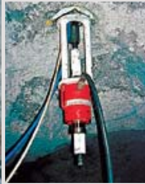
Underground installation team; Small picture: Stressing operation with local jacks using a stressing chair
