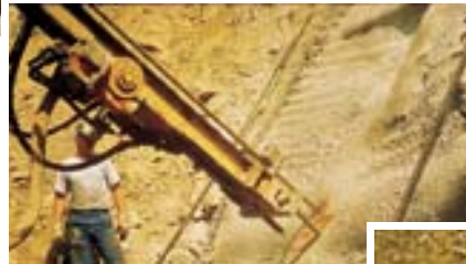
Drilling with anchor rods
