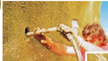
Grouting through hollow core
