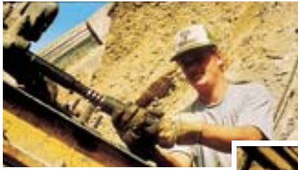
Connecting the drill bit
