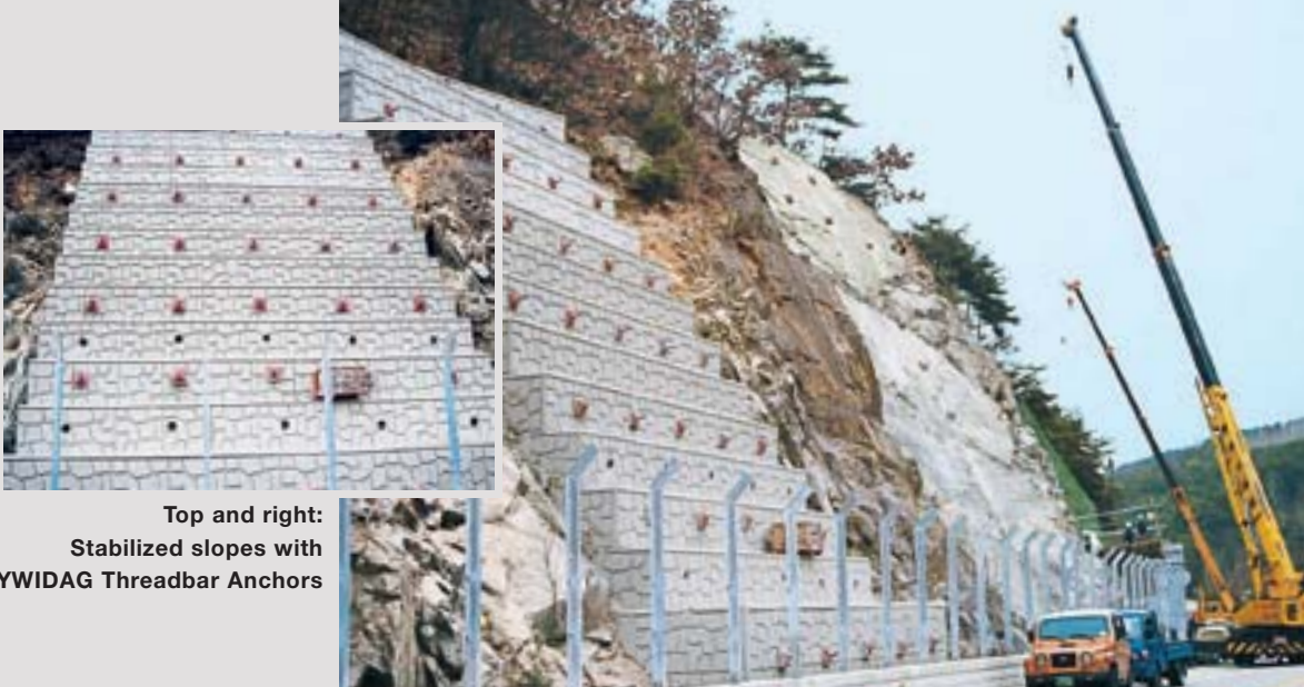
Slopes secured with DYWIDAG Threadbar Anchors
