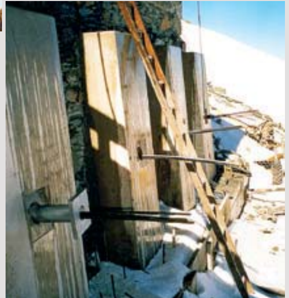
DYWIDAG Strand Anchor after installation
