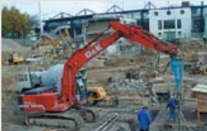
i Project Sports Facility Linz, Austria +++ Client Structural analysis: Kirsch-Muchitsch & Partner +++ Owner Town of Linz DSI Services 1,200 m of Ø 170 mm grouted DYWIDAG Ductile iron piles; foundation of pillars 10 m.
