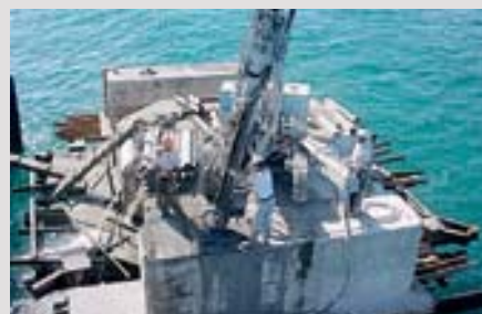
Installation of DYWIDAG Micropiles Ø 57 mm, between 37 and 42 m long
