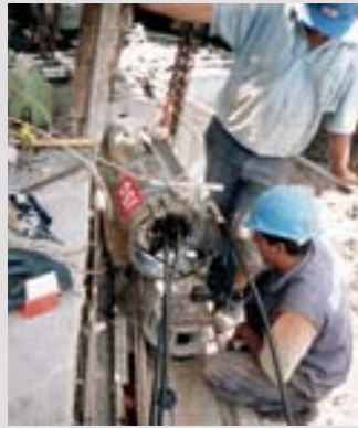
Prestressing tests performed on the anchors
