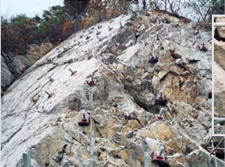
Slopes secured with DYWIDAG Threadbar Anchors
