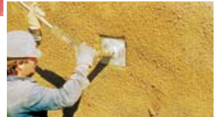
Stressing the anchor by torque wrench or hollow cylinders
