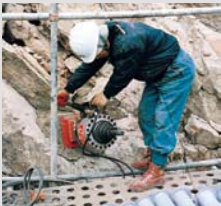
Stressing of the anchor with DYWIDAG Jack
