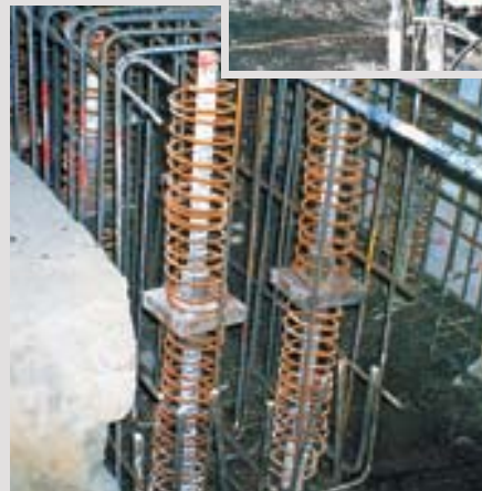
Detail view of GEWI® Pile head (compression/tension)
