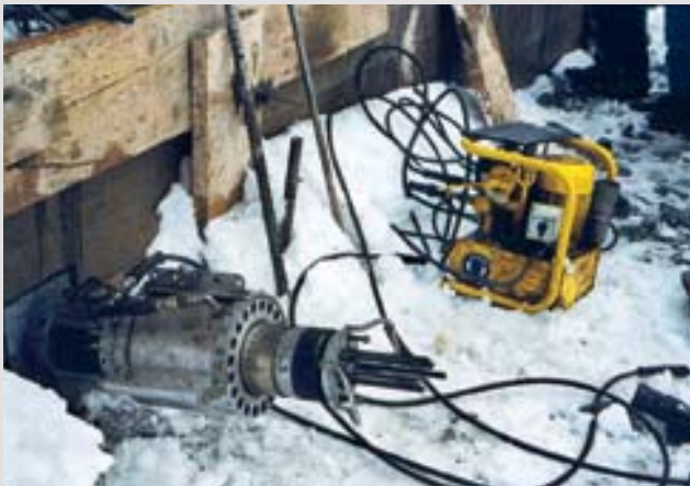
Tensioning of the DYWIDAG Strand Anchors
