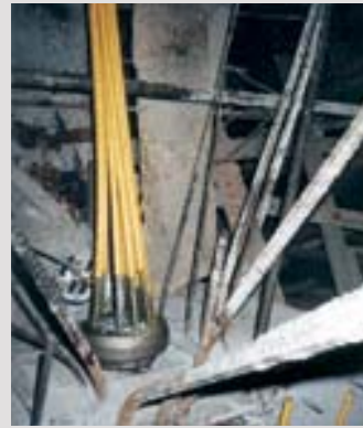
Lengthening of anchors with couplers of type R
