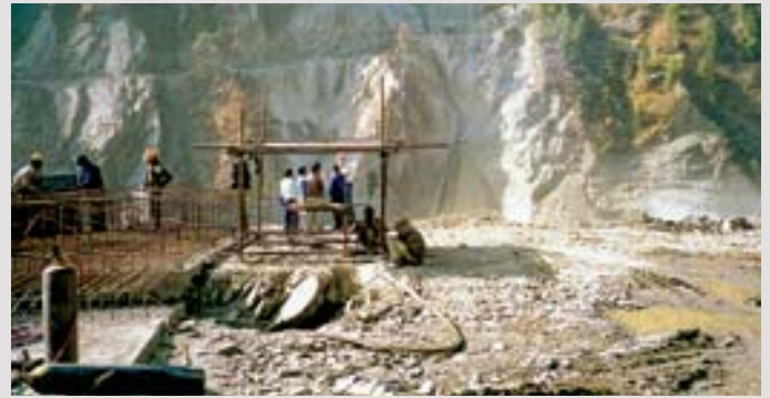
Position of the concrete dam with foundation for cable cranes
