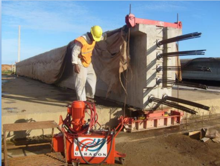
Shifting of PC Girders
