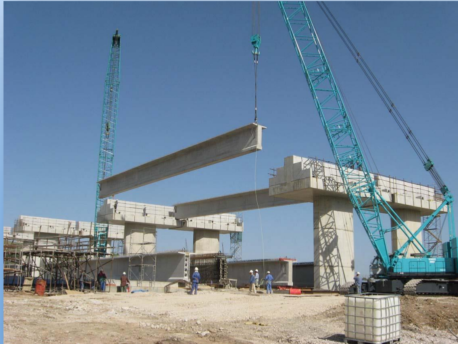
Erection of PC Girders
