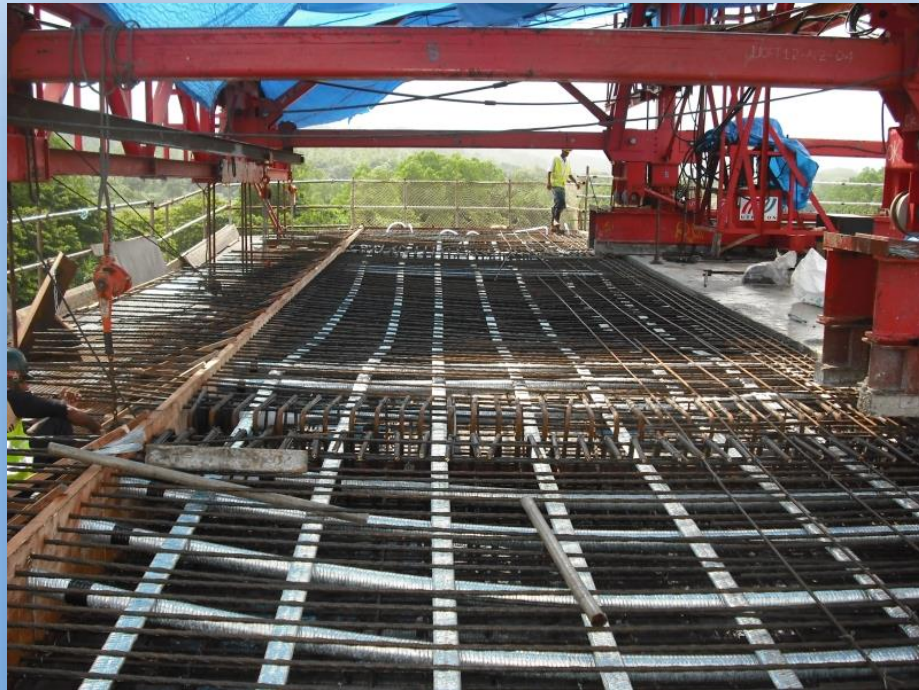
Longitudinal and Transverse Tendon Layout
