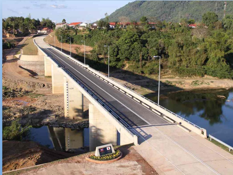
Hinheup Bridge, Laos
