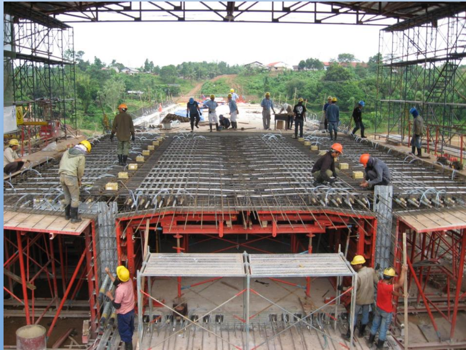
Hinheup Bridge, Laos
