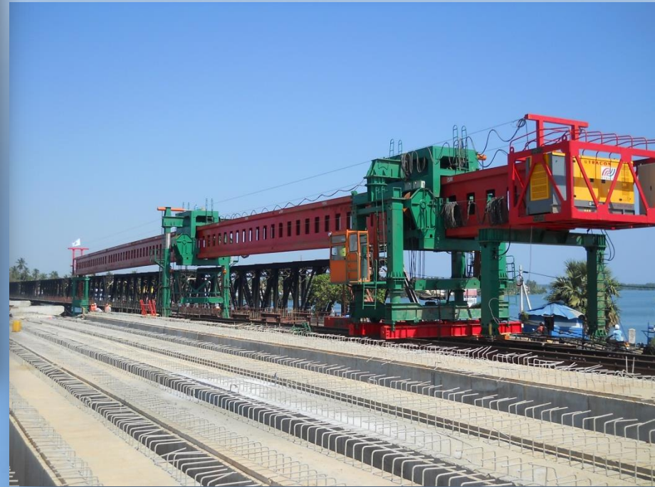
Setting up of Beam Erector
