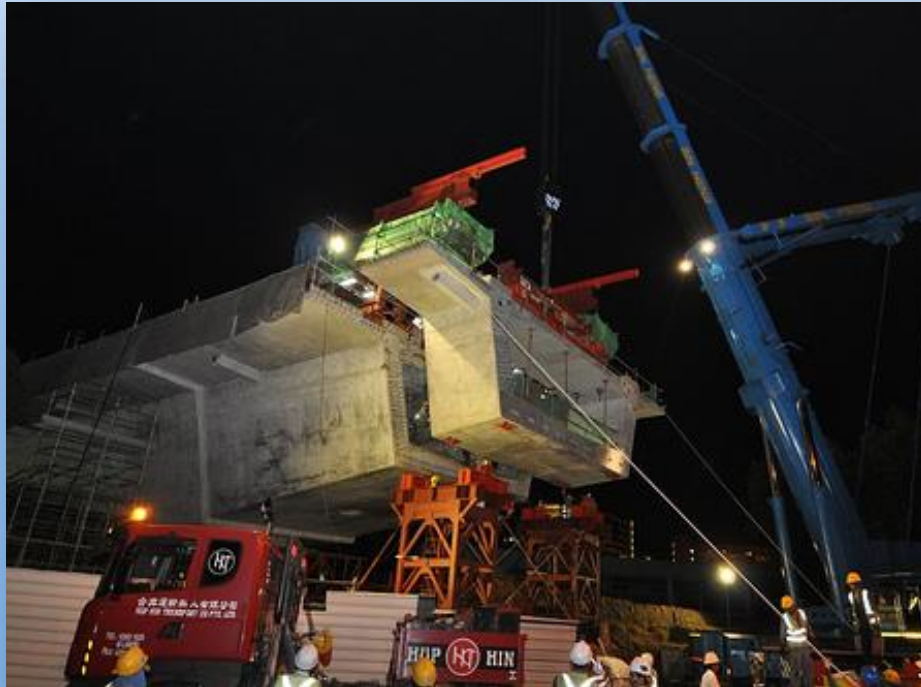
Installation of Starter Segment
