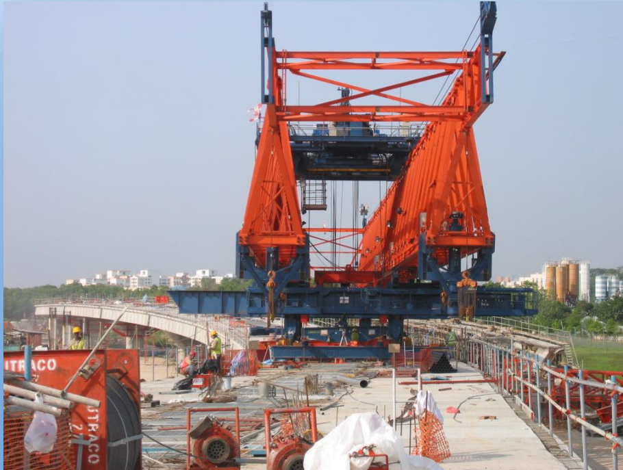
Reverse Walking of Launcher
