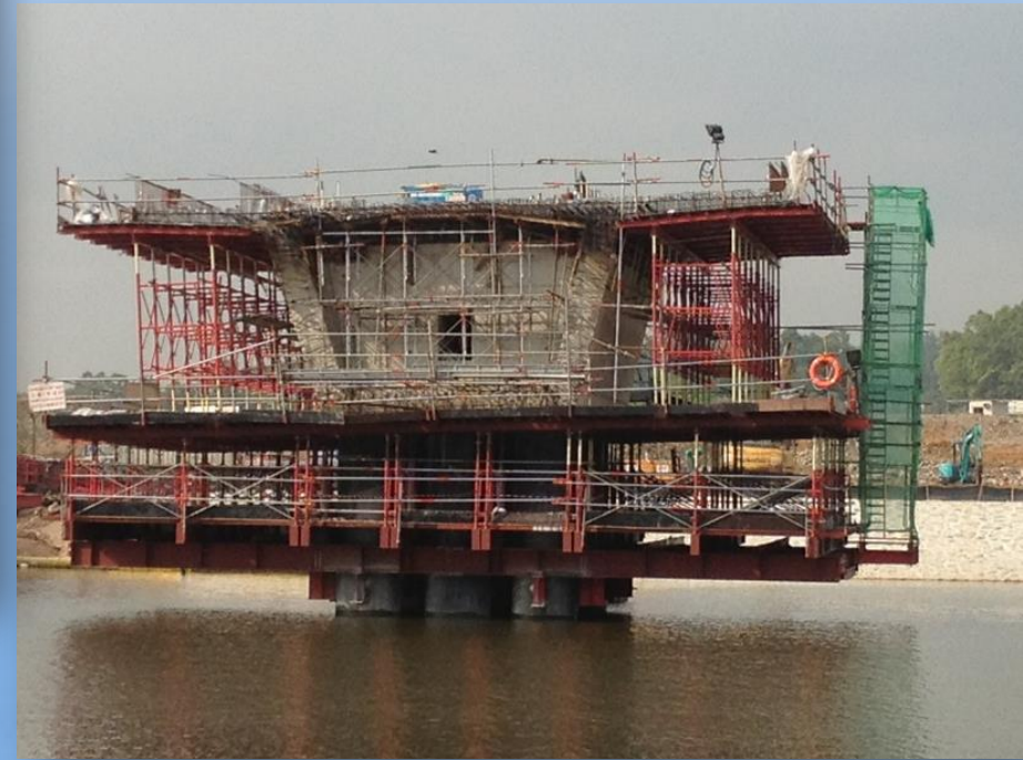
Pier Table Construction
