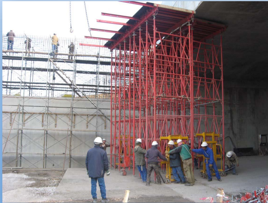
Tunnel Slab Construction
