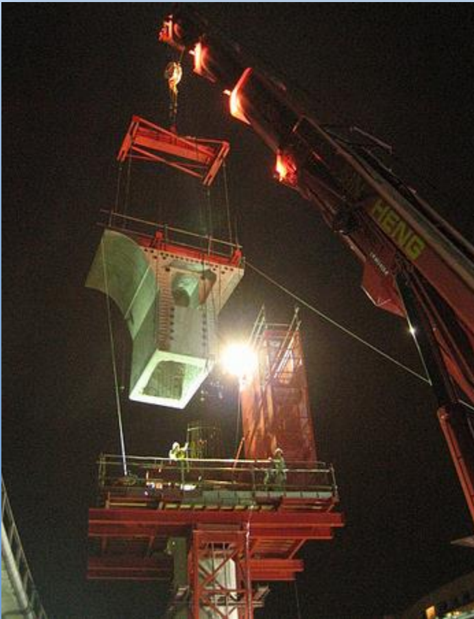
Installation of Pier Segment
