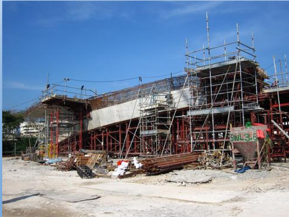
Precasting in Operation
