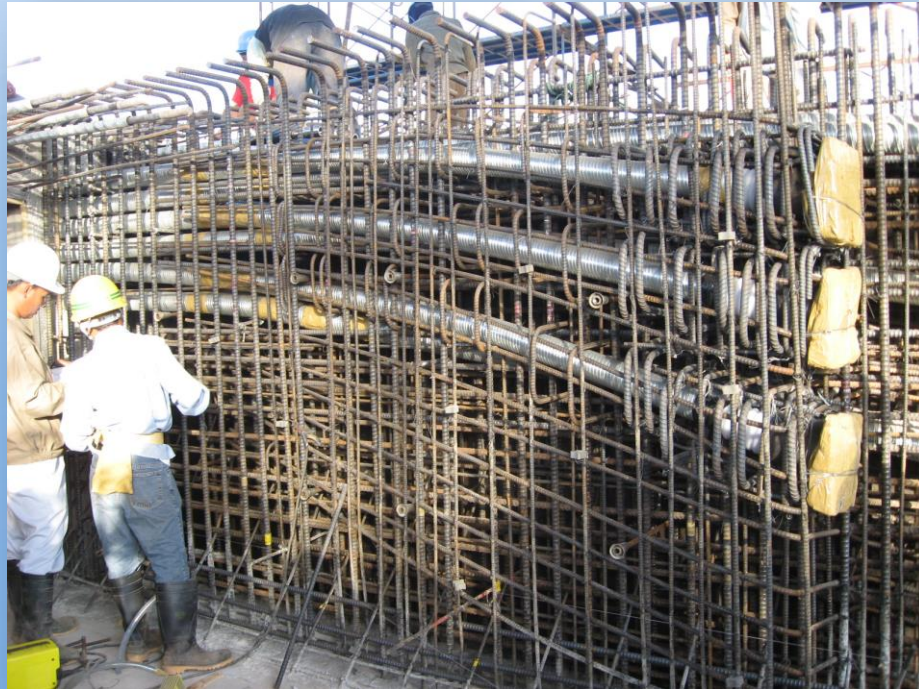
Hinheup Bridge, Laos
