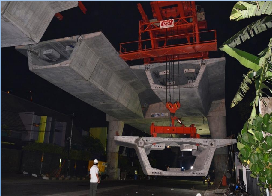
Segment Lifting in Operation
