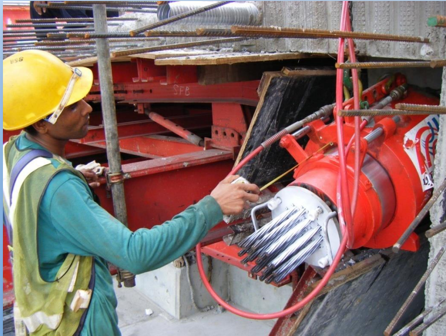
Prestressing of Cantilever Tendons
