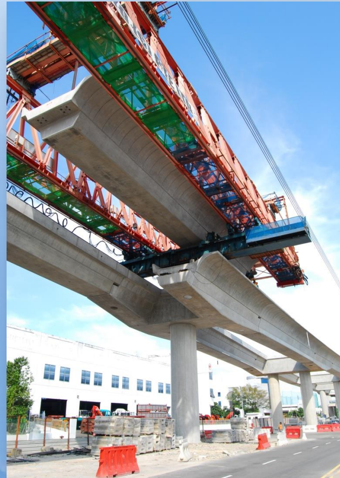
Full Span Erection by Overhead Launcher
