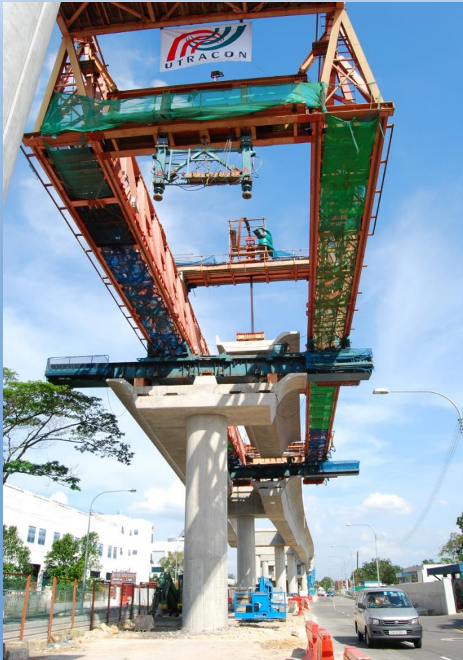
Full Span Erection by Overhead Launcher
