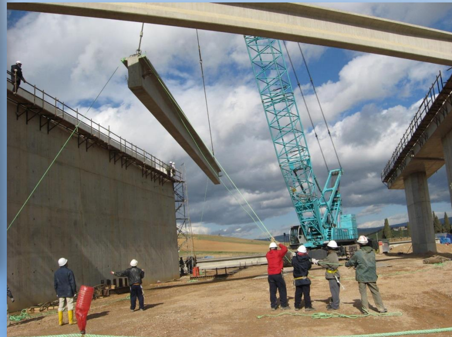
Erection of PC Girders
