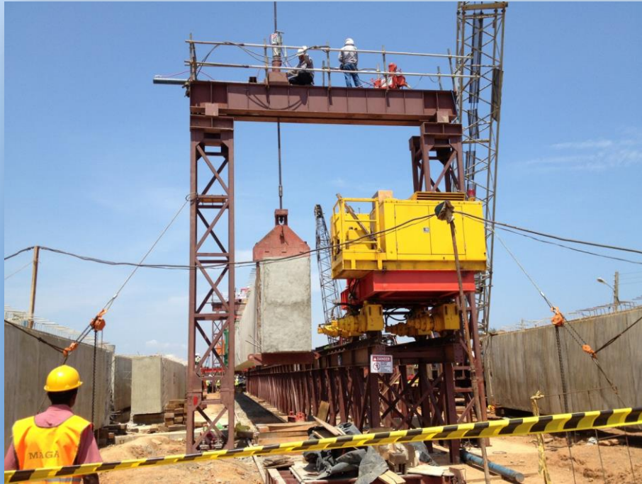
180-ton Capacity Loading Facility
