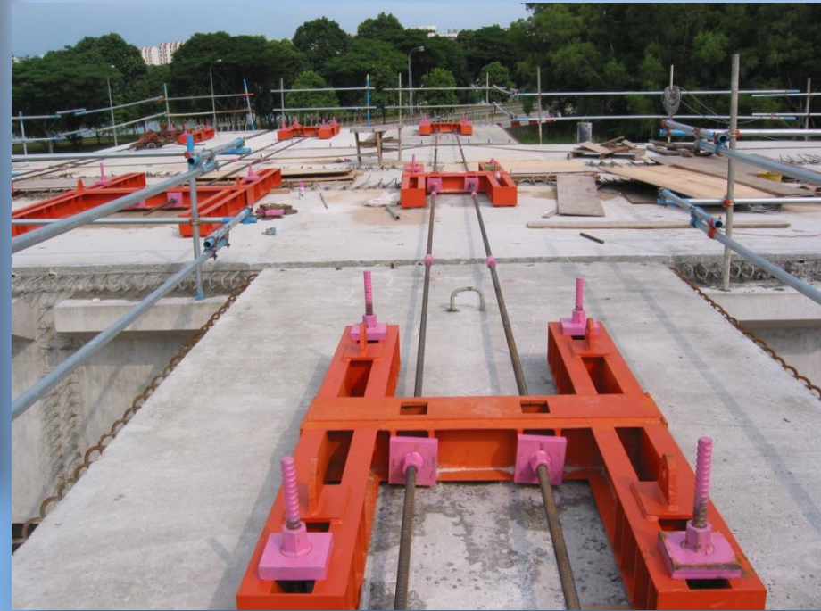
Temporary Holding of Wing Segments
