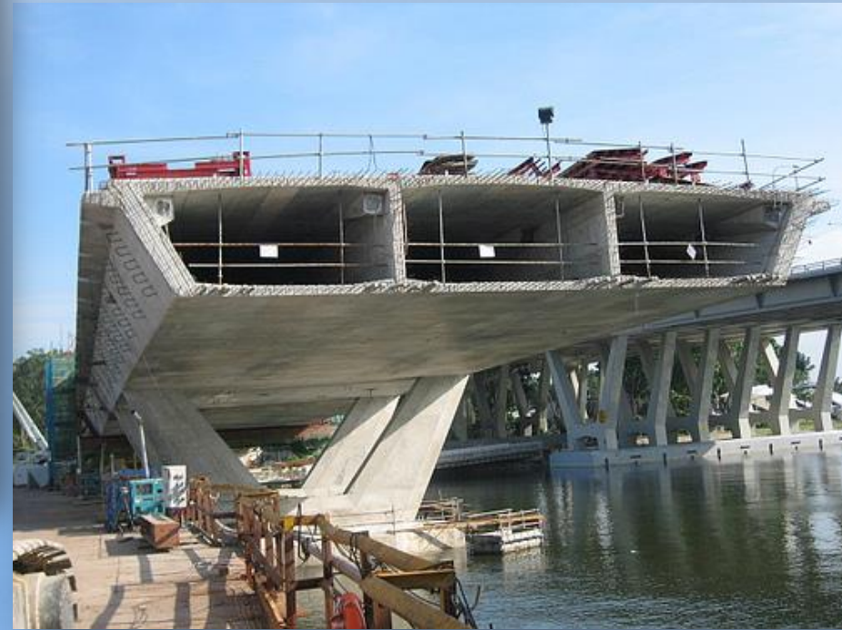
Completed Cantilever
