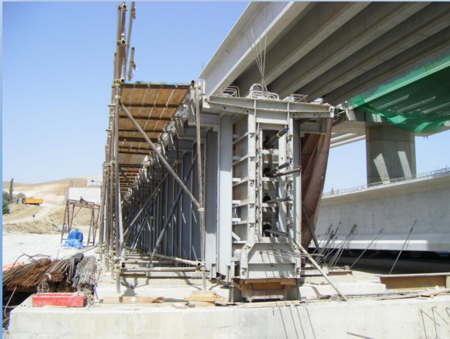
Mould for Precast Girder
