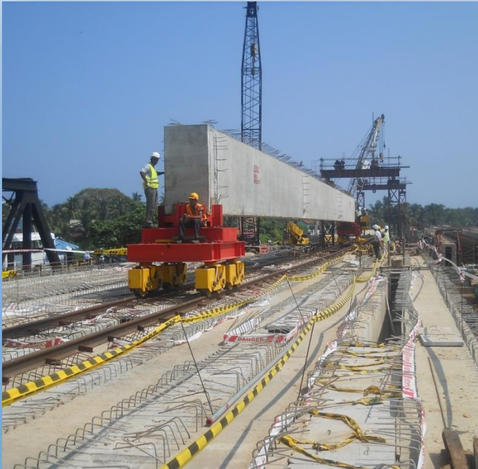
Transportation of temporary rail
