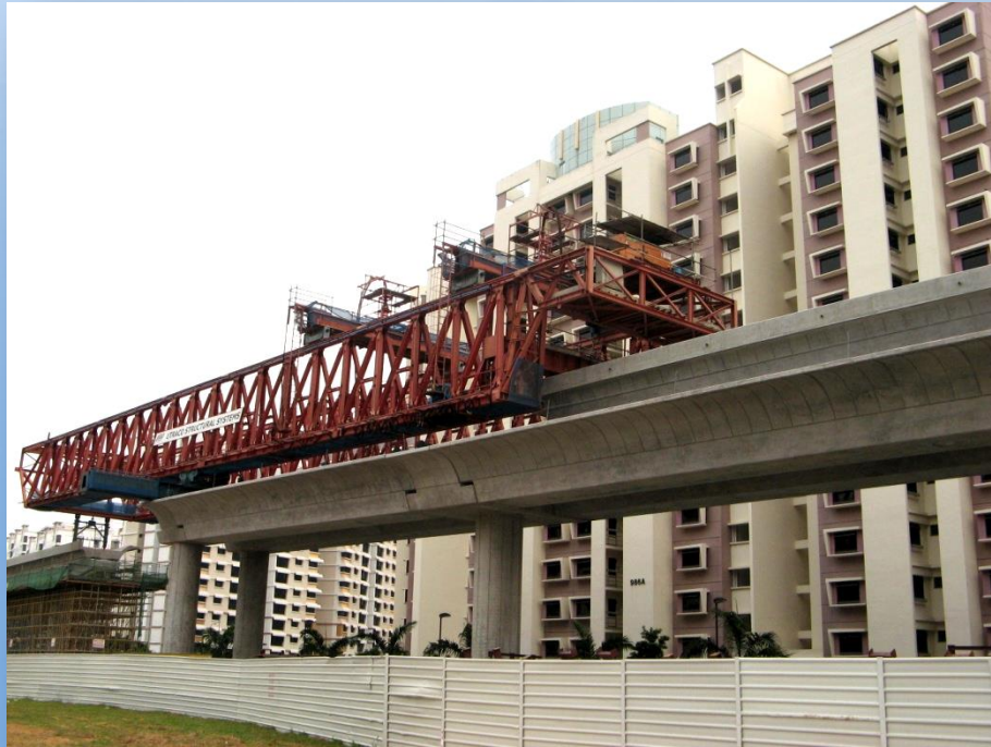
Launching of Launcher
