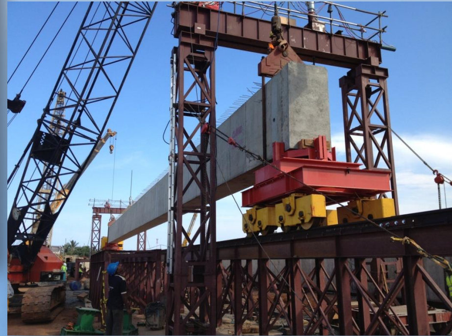
Lifting of Precast Girders
