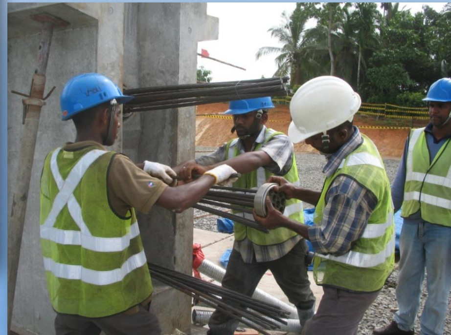
Wedge Plate Installation
