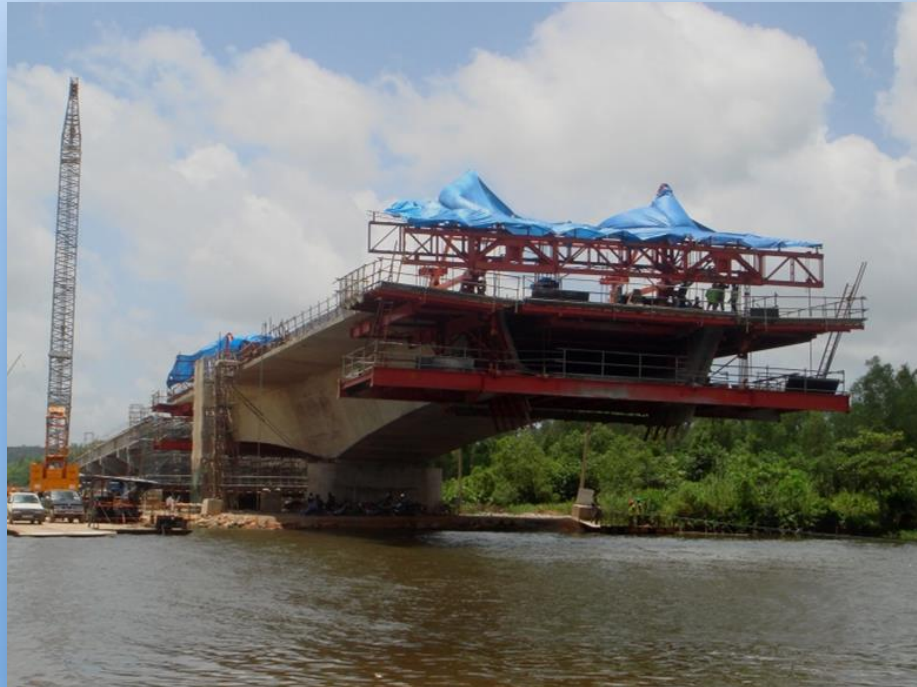
Cantilever Construction using Form Traveller
