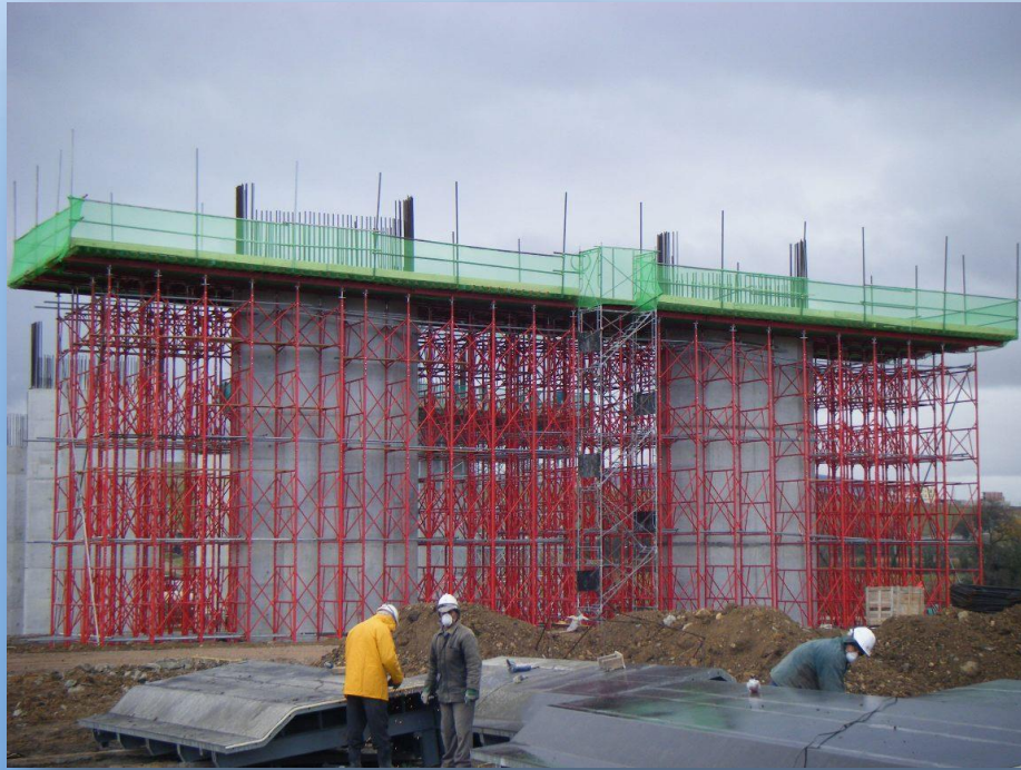
Crosshead Construction
