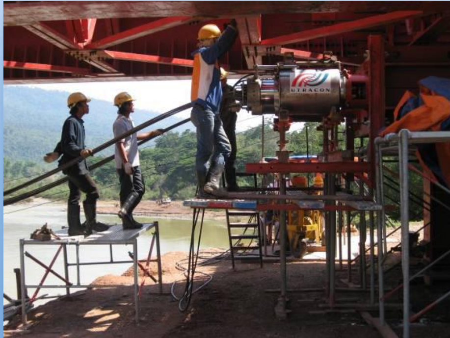
Hinheup Bridge, Laos
