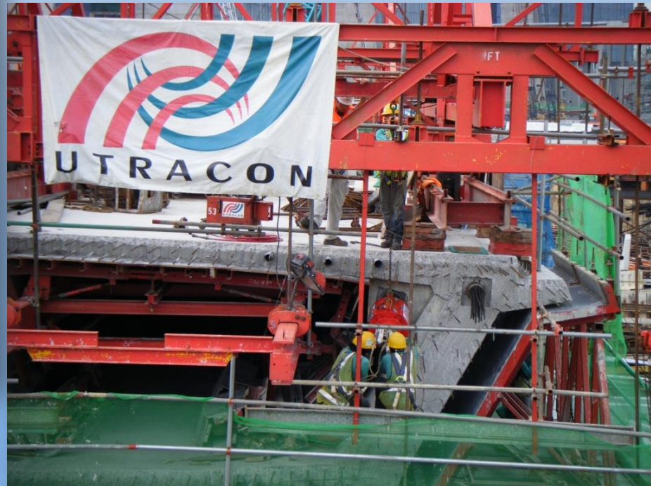
Prestressing of Cantilever Tendons
