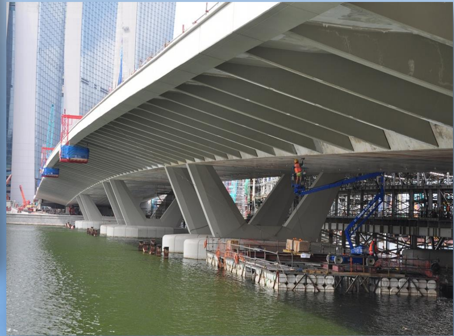
Marina Bay Bridge, Singapore
