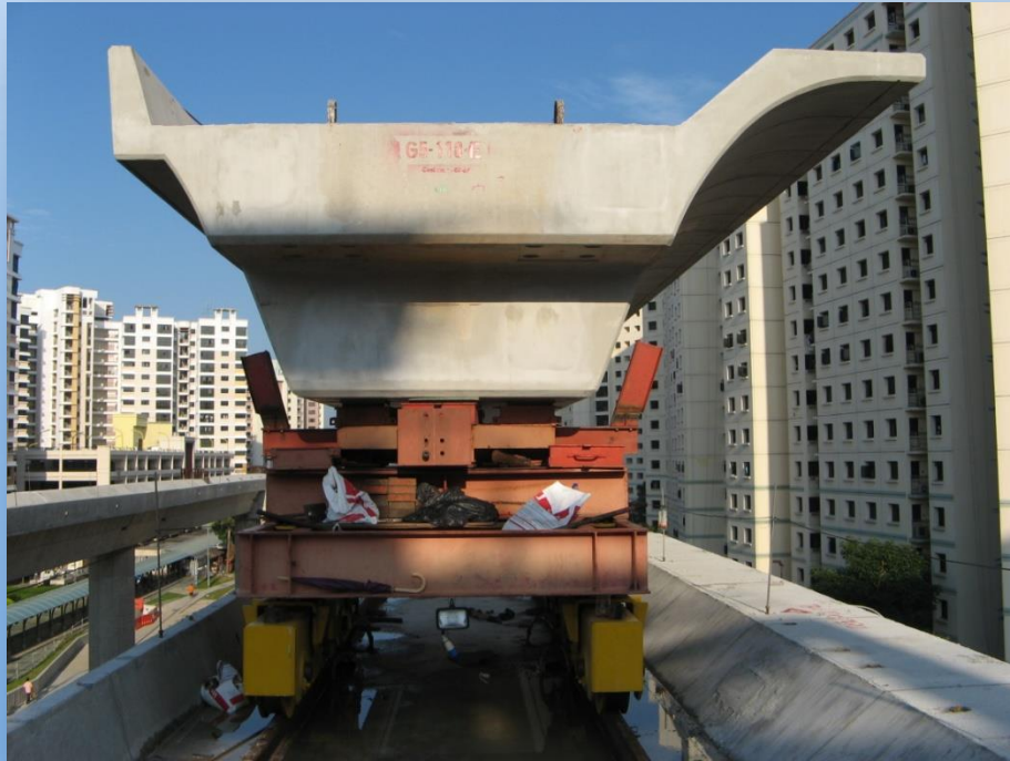
Delivery on Erected Spans
