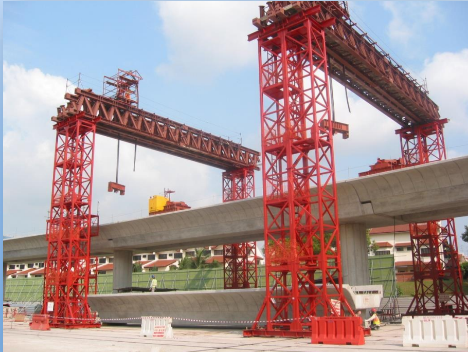
300-ton Capacity Loading Facility
