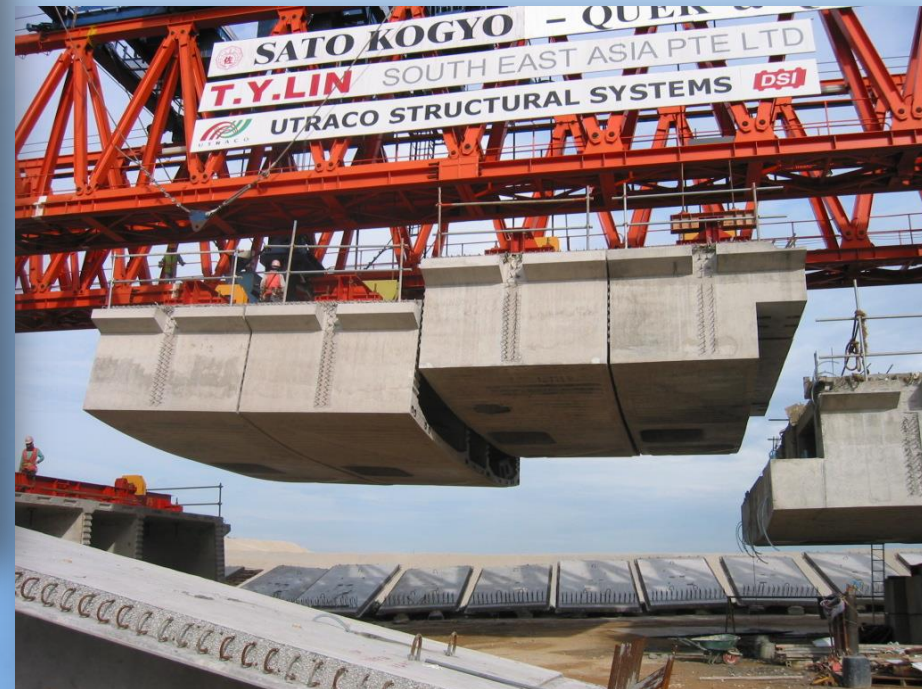
Arrangement of Precast Segments
