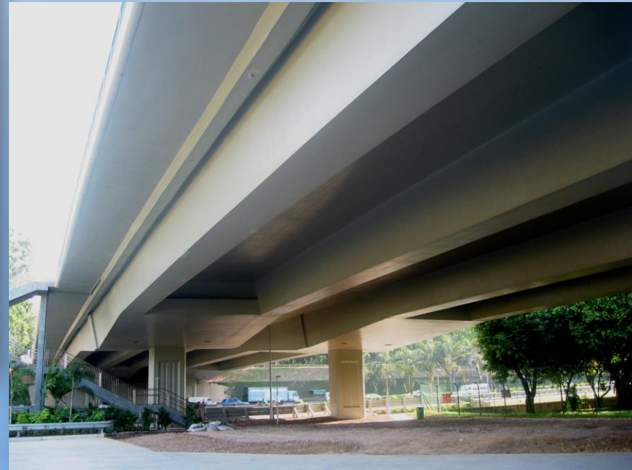
PC Girders Erected
