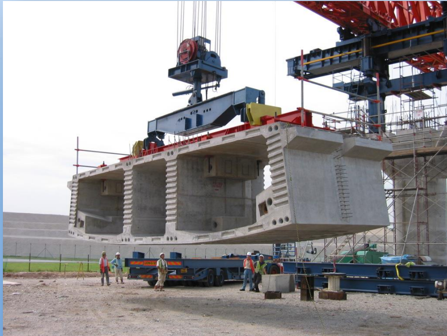
Lifting of 60 - 90 ton Precast Segments
