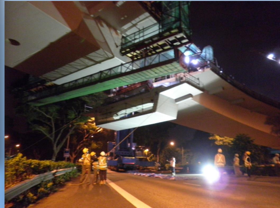
Installation of Cantilever Segment
