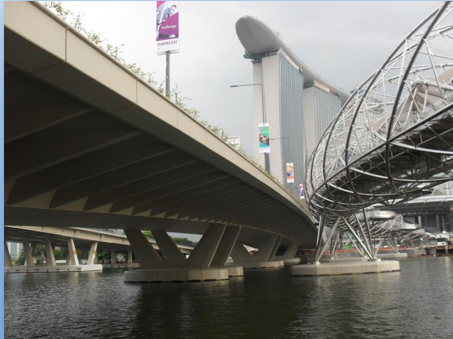
Marina Bay Bridge, Singapore
