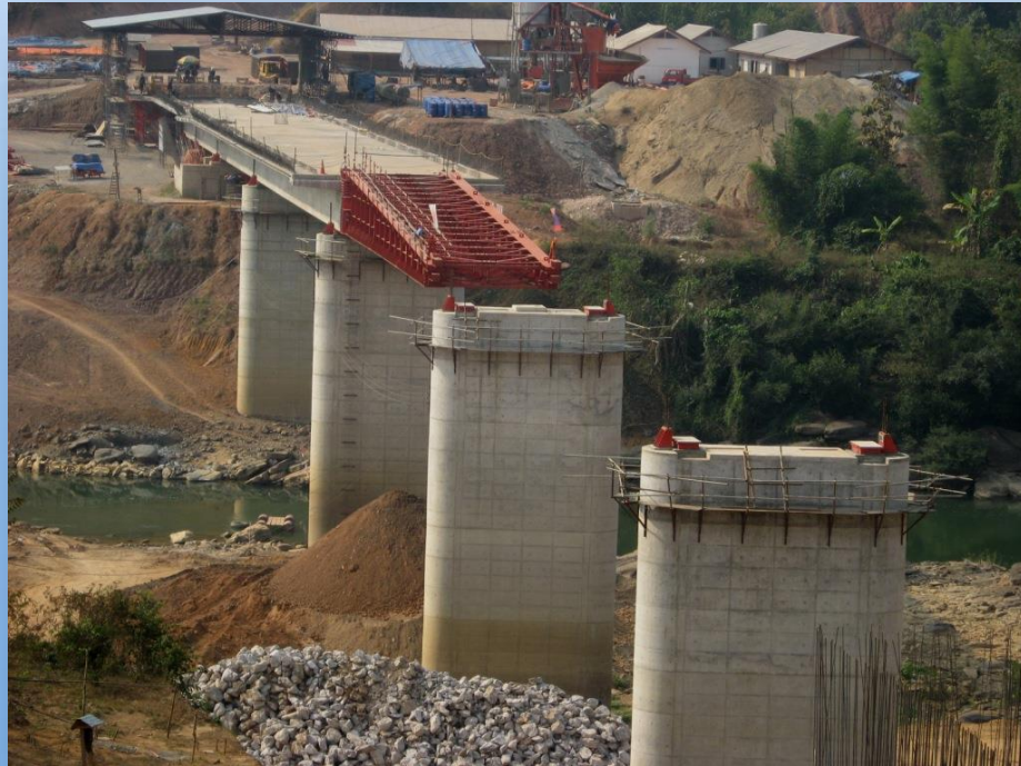
Hinheup Bridge, Laos
