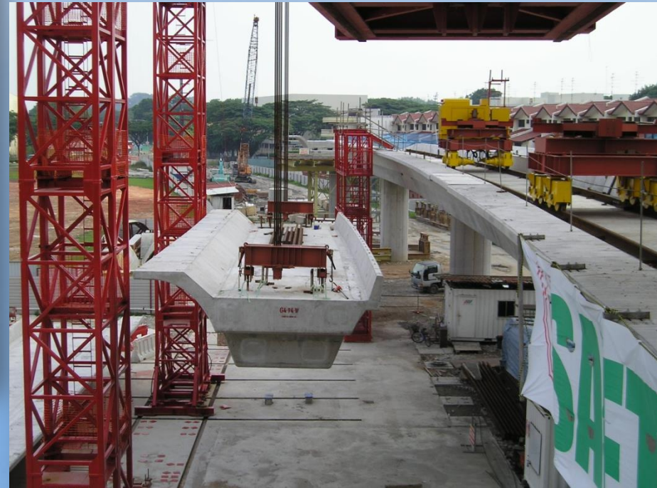
Lifting of Precast Girders
