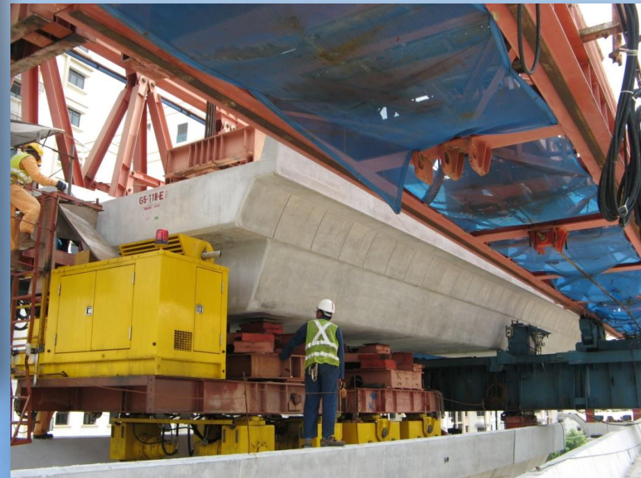
Placement of Precast Beam
