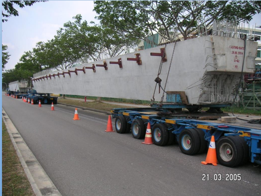
Delivery of PC Girders
