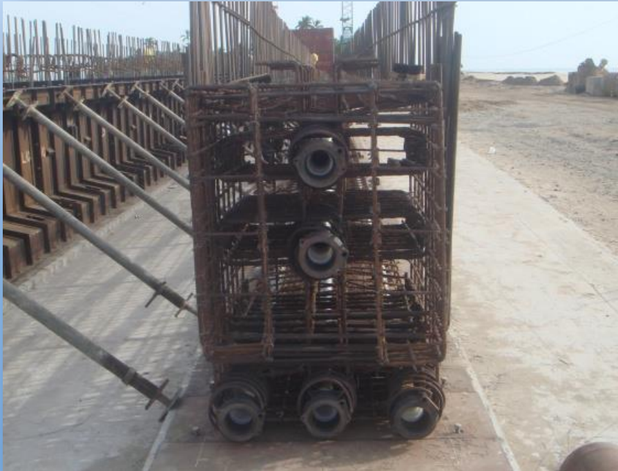
Installation of Anchorages
