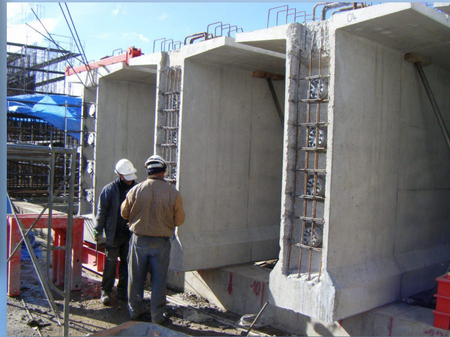
Completed Precast Girder
