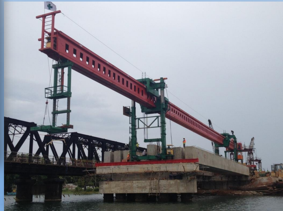
Positioning of Beam Erector
