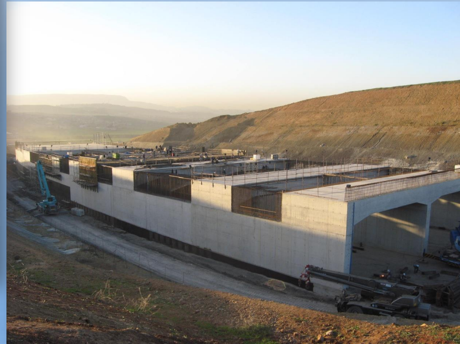
Partially Completed Tunnel
