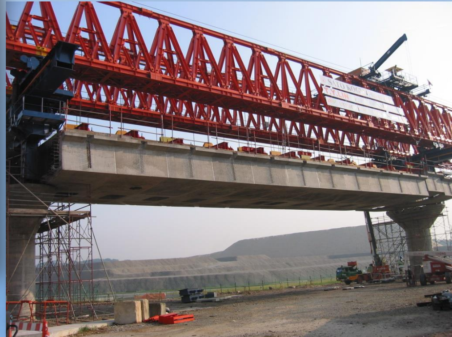
1000-ton Capacity Launcher
