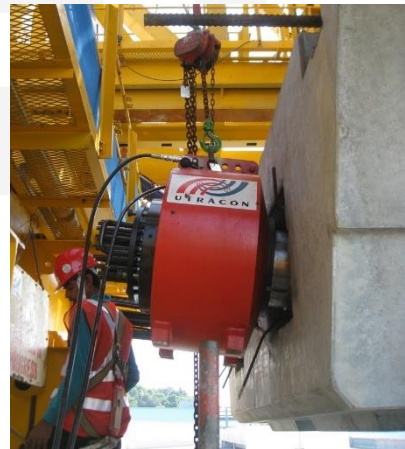
Full span stressing before lowering
