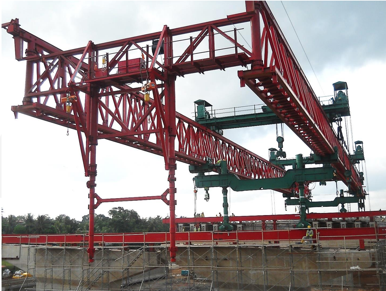
Slim supports, widely spaced truss
