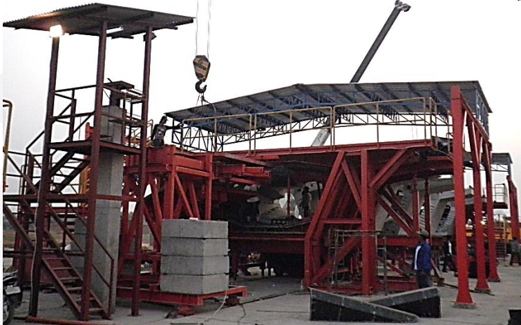
GC during precasting
