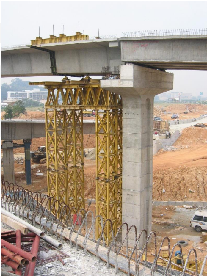
Shoring for end span segments
