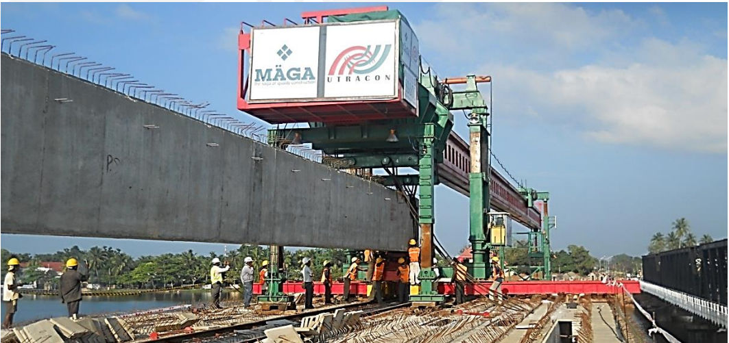
Delivery of girder by locomotive and railcar on temporary railway
