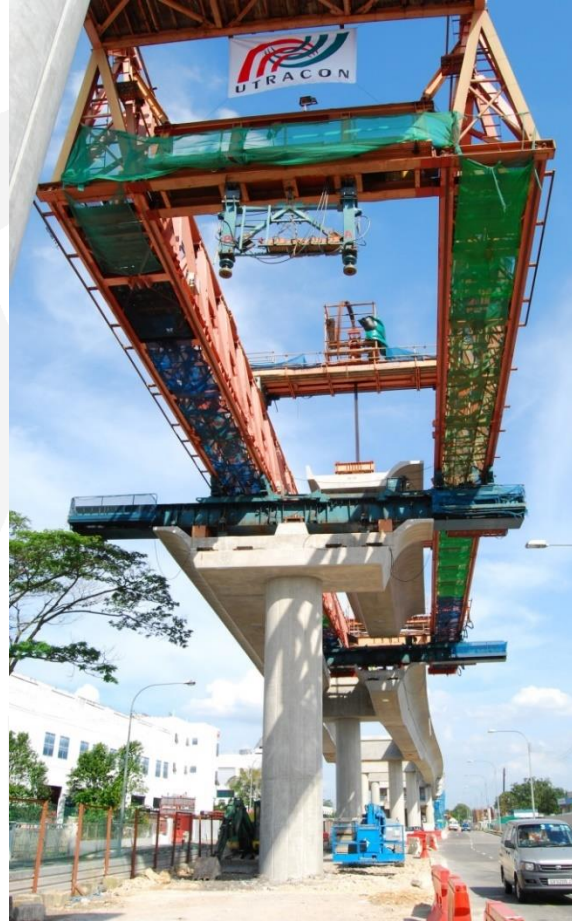
Full span girder for Singapore MRT – maximum 270 ton
