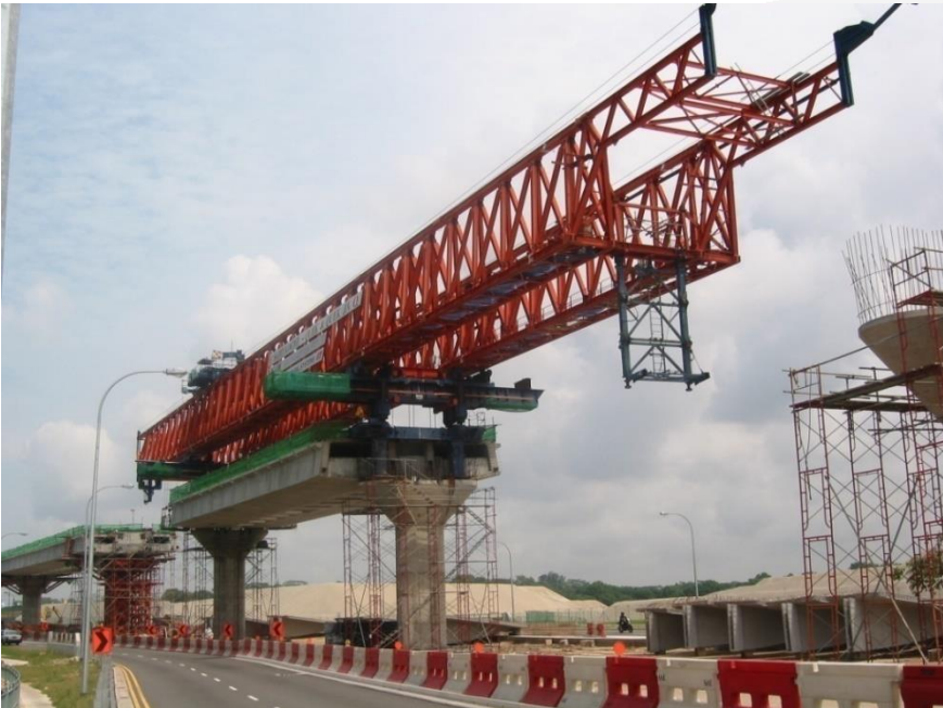
LG's supports on pier heads
