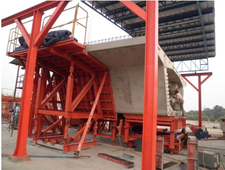
Segment casting yard
