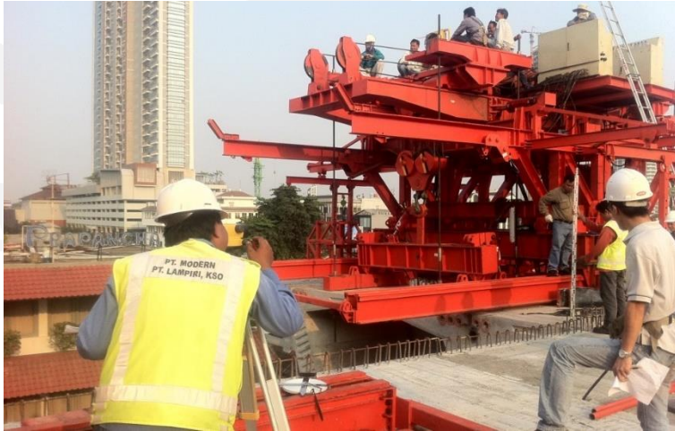
GC during erection
