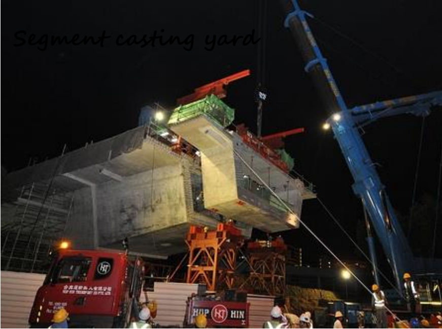
Launching of cantilever segment
