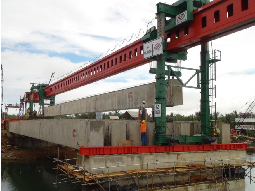
Launching of precast girder
