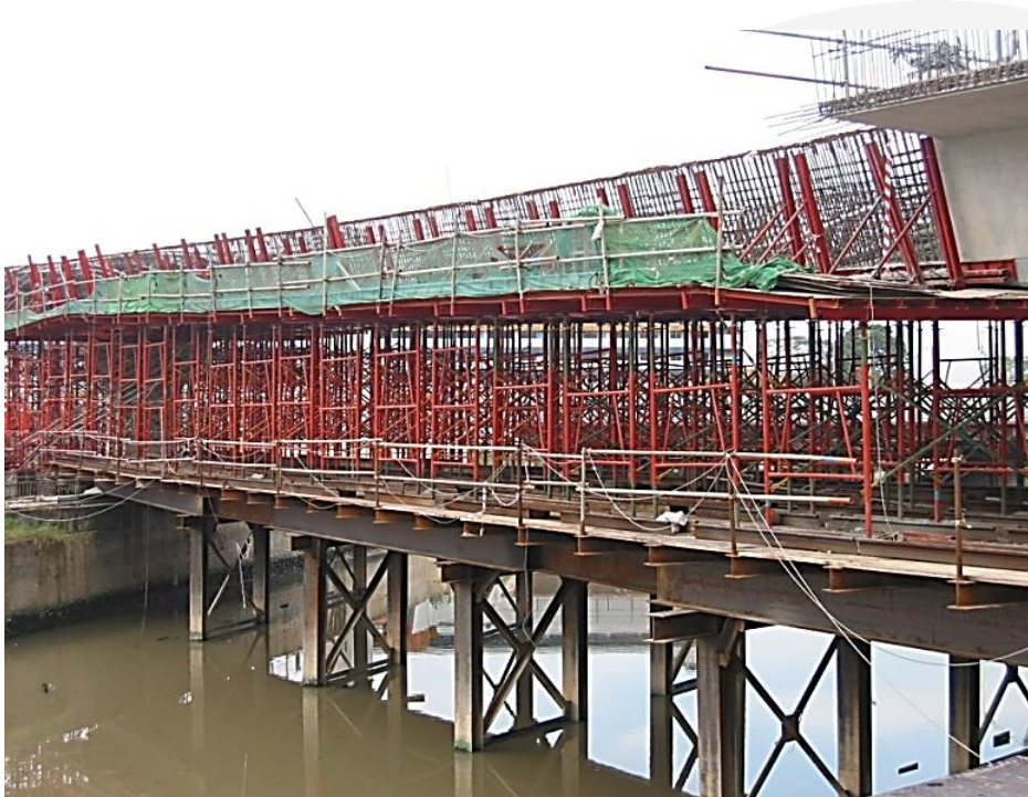
Staging onto river bed
