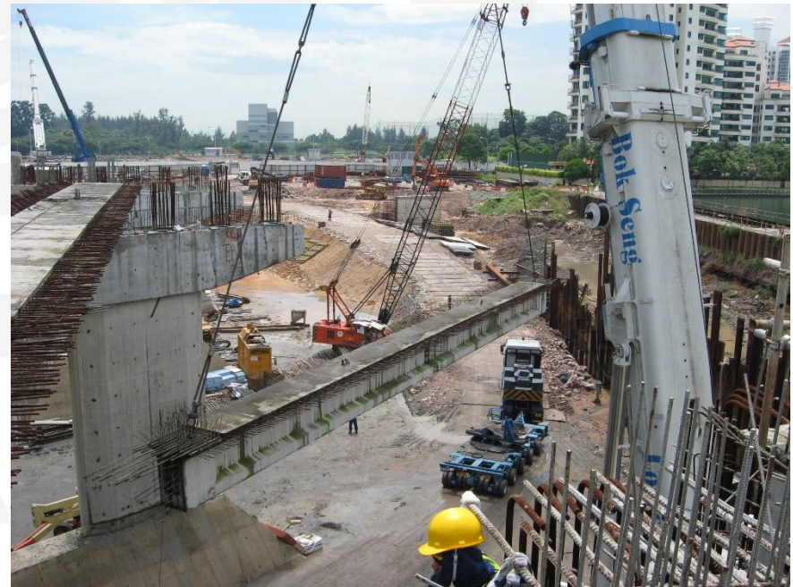
Single crane lifting
