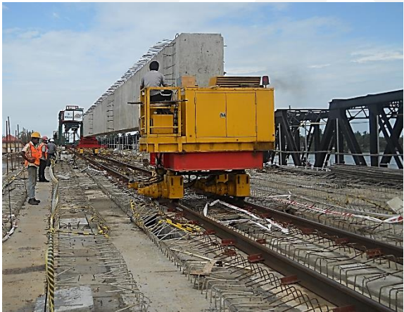
Delivery of girder by locomotive and railcar on temporary railway
