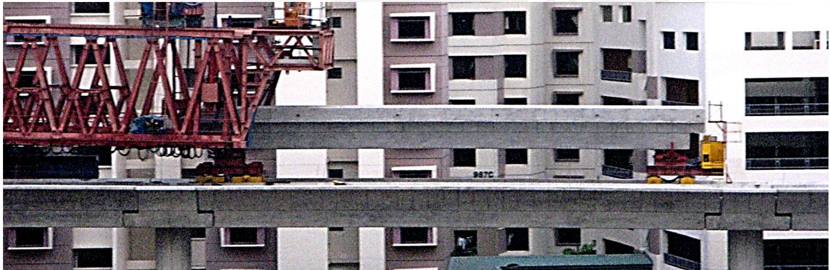
Launching of truss using PC girders as counterweight
