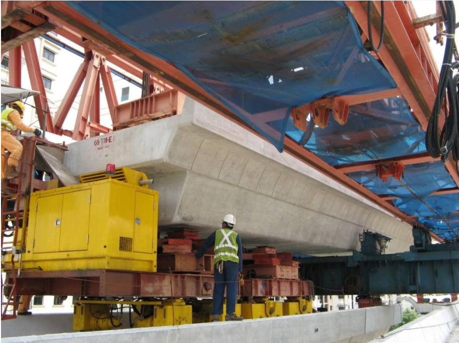
Feeding in of full span girder
