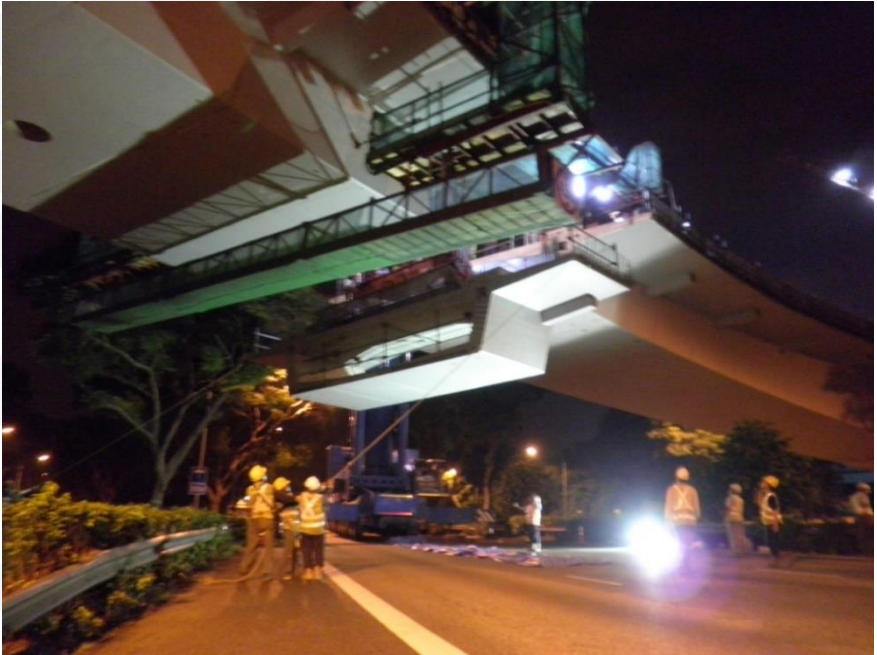
Launching of closure segment
