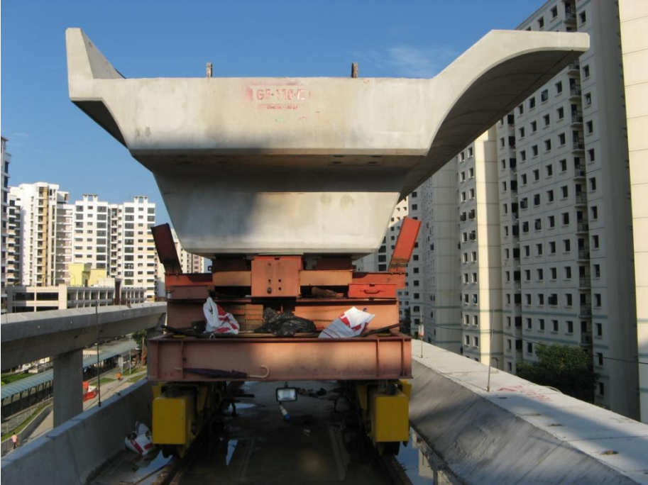
Transporting girders on erected decks
