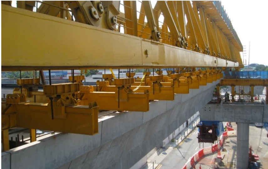
Full span stressing before lowering
