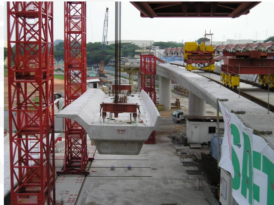
Uploading of full span girder
