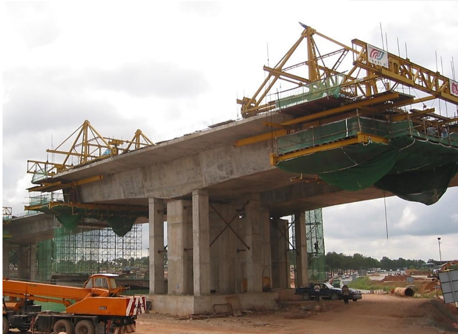
Stabilising with fictitious columns
