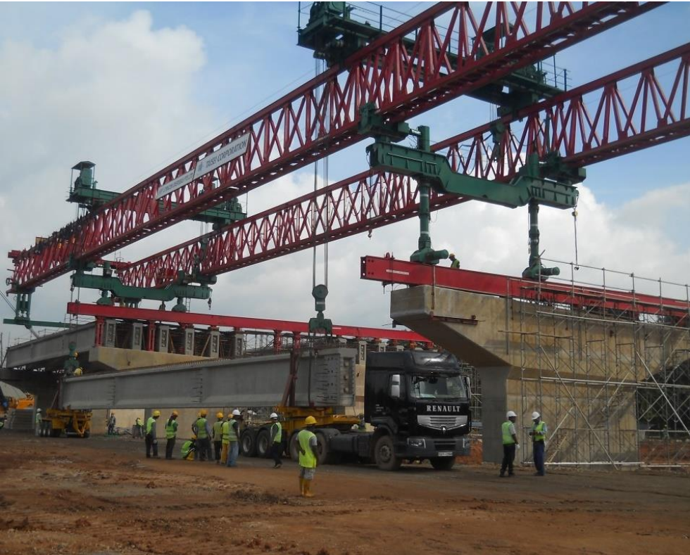
Lifting of girders from the side
