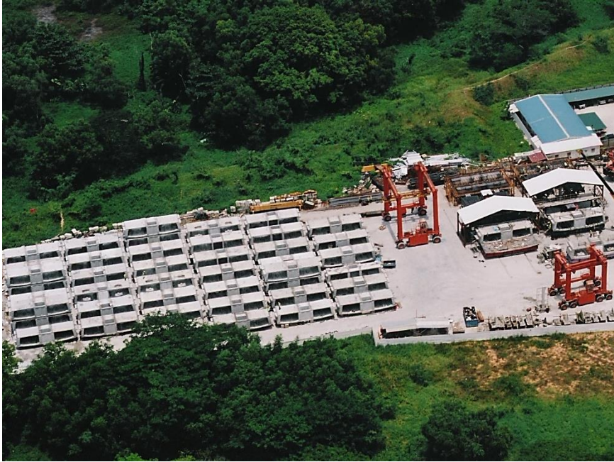
Segment storage yard
