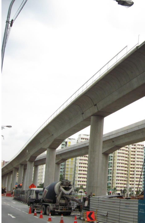
Full span girder for Singapore MRT – maximum 270 ton
