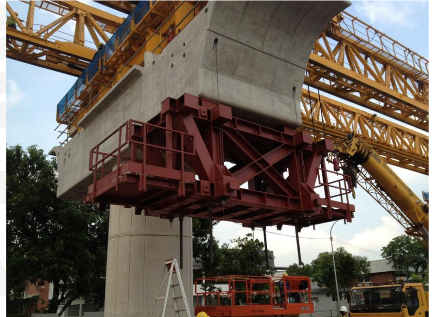
Erected span rested on temporary support while being stitched
