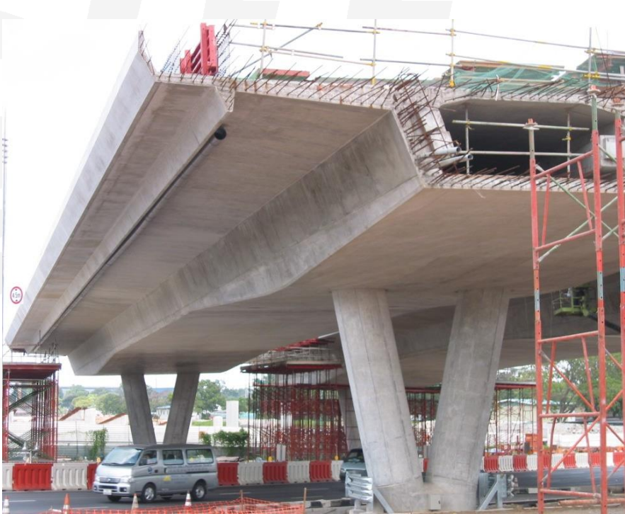
Traffic diversion is required
