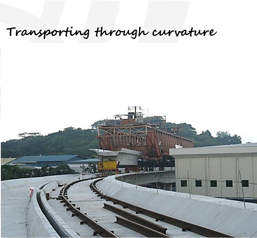
Transporting girders on erected decks
