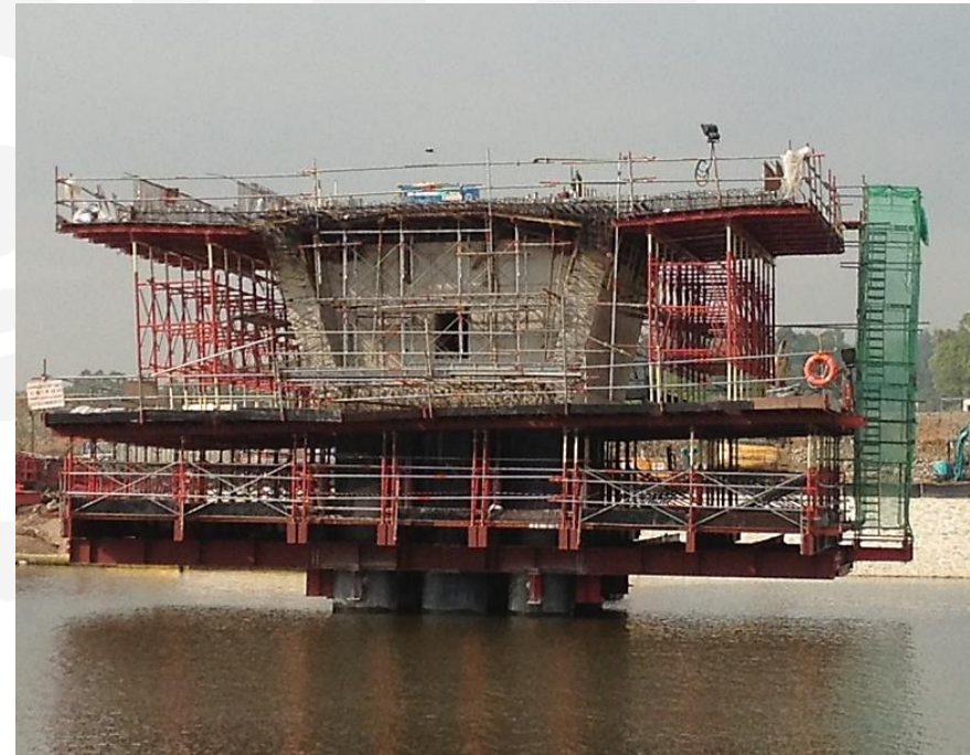
Staging supported by piers
