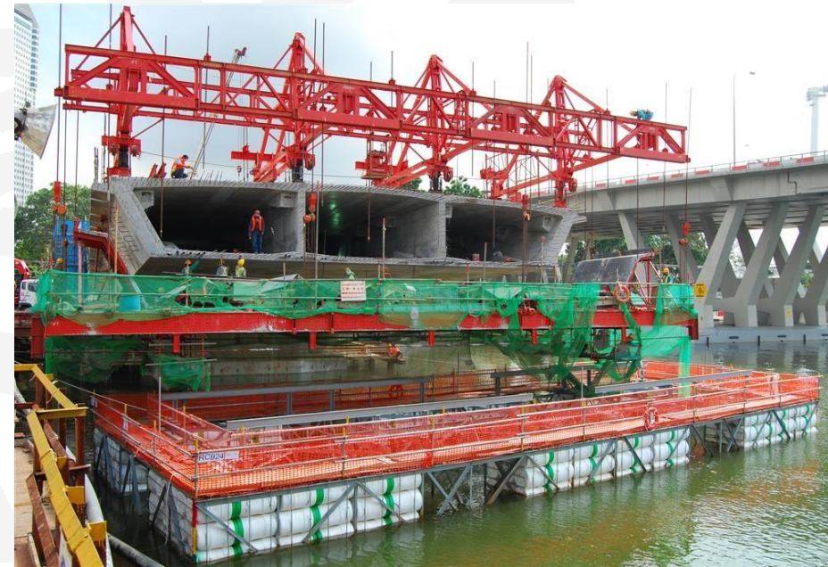
Lowering bottom platform onto pontoon
