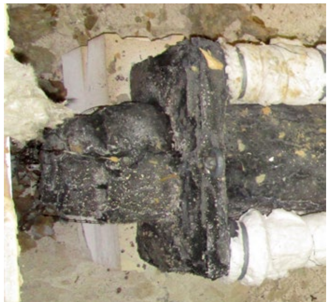
Intumescent Coating after Fire Testing
