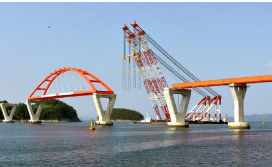
Gajo Arch Bridge, South Korea 80 Type DG-P 12 DYNA Grip® Hangers
