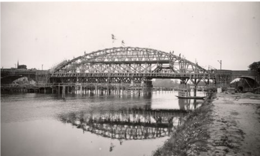
1928: Saalebridge, Alsleben, Germany First Bridge with prestressed Beam Tie developed by Dr.-Ing. Franz Dischinger
