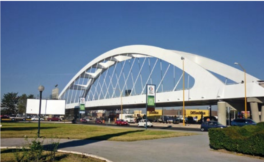
Aguascalientes Arch Bridge, Mexico Supply and installation of 34 Type DG-P 19 DYNA Grip® Hangers
