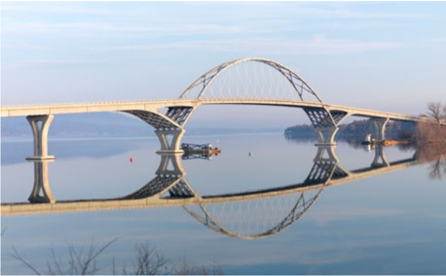
Lake Champlain Arch Bridge, USA Design, supply and installation of 64 Type DG-P 7 DYNA Grip® Hangers
