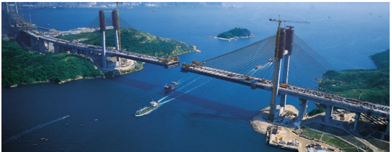
1995: Kap Shui Mun Bridge, Hongkong, China DYNA Bond® Stay Cable Bridge with 176 cables
