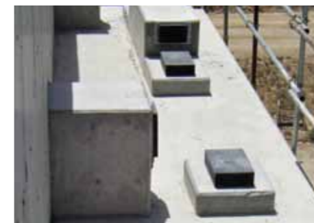
Elastomeric Bearing
