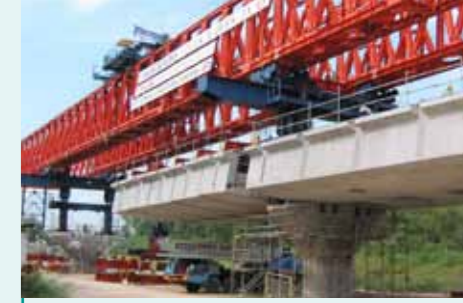
Span-by-Span Method
