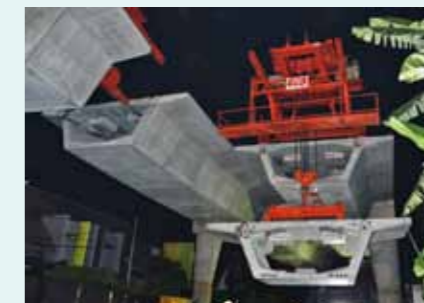
Cantilever Segment Erection
