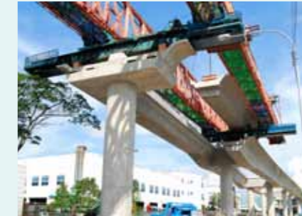
Full Span Launching
