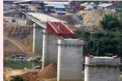
ILM for Concrete Bridge
