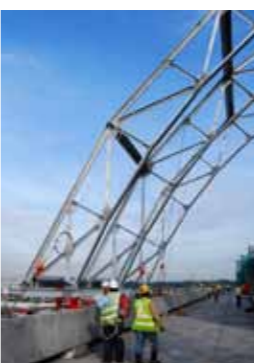
Roof Truss Sliding
