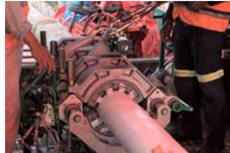
Stay Duct Welding
