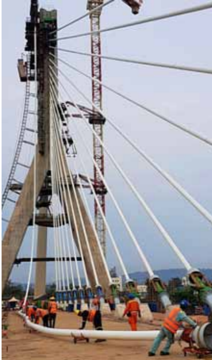
Stay Duct Installation
