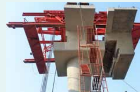
EJ Segment Erection
