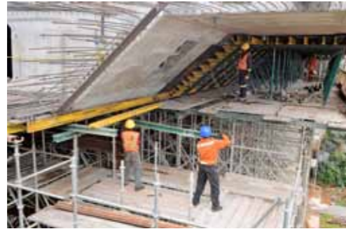
Box Girder Formwork
