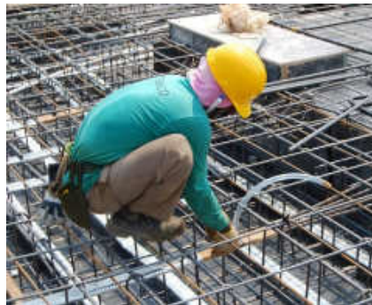
Fixing of grout vent / hose
