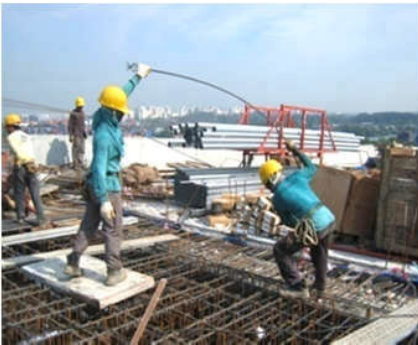
Laying of beam tendons
