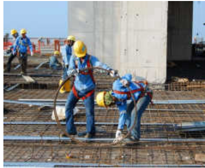
Uncoiling of precut strands
