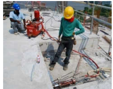
Stressing of slab tendon
