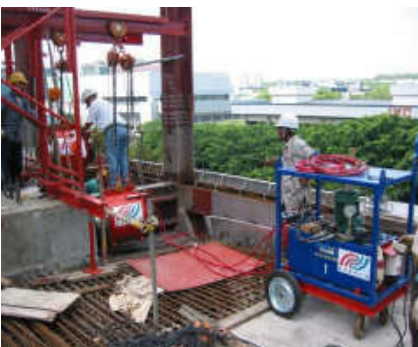
Stressing of beam tendon
