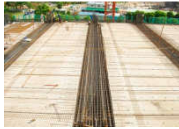
PT beam with PC slab
