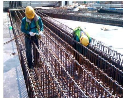
Fixing of beam tendon support bar
