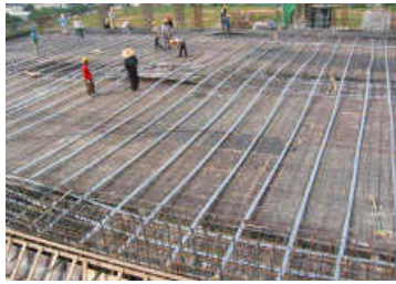
PT beam & slab
