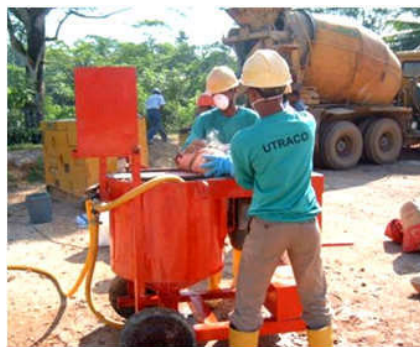
Mixing of grout for tendon grouting
