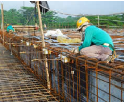
Fixing of slab anchorages
