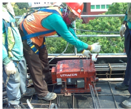
Installation via strand pusher
