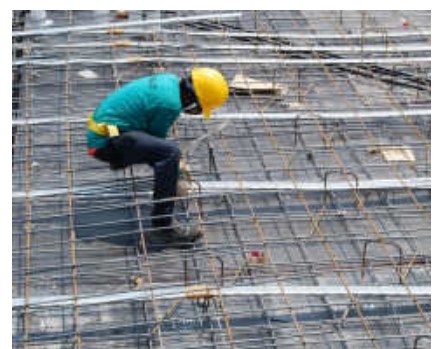
Fixing of slab tendon bar chair
